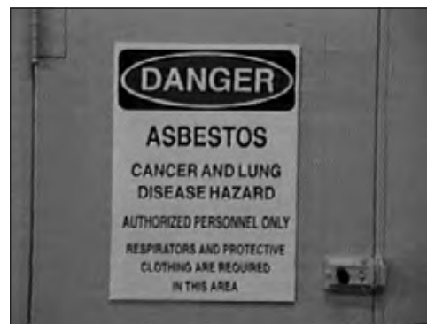
Warning Sign Outside of Asbestos Work Being Conducted in a Boiler Room
